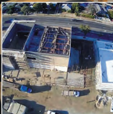
St. Genevieve Parish Hall and Performing Arts Center under construction
