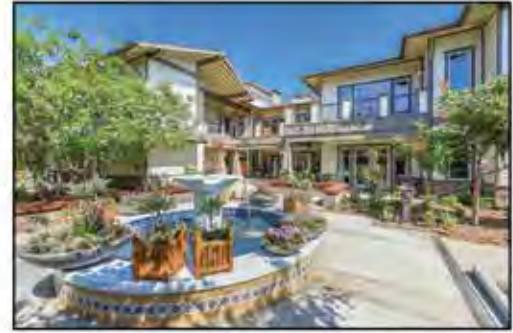
Santa Teresita Cottage Construction
