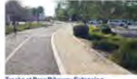
Tracks at Brea Bikeway Extension
